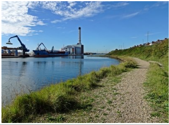
Westwards: the power station
